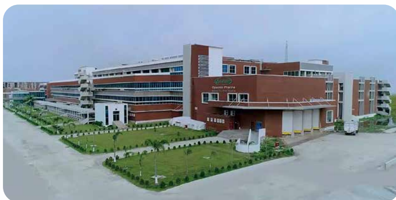
Bank Asia financed pharmaceutical production facility of Opsonin Pharma Limited
