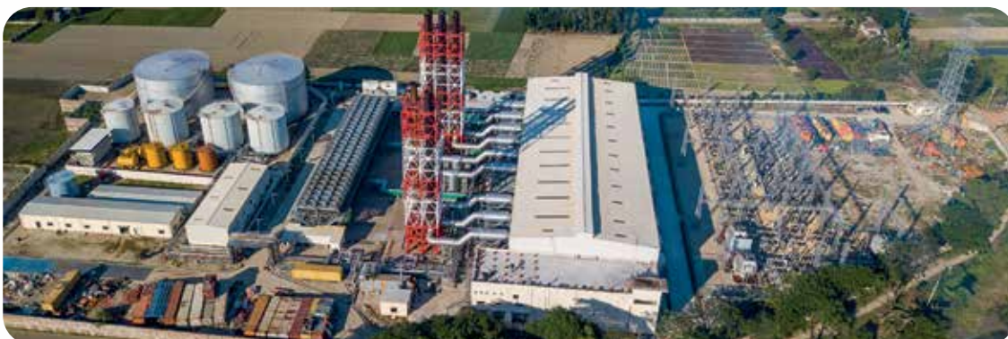
54.50 MW power generation facility of Bhairab Power Limited
