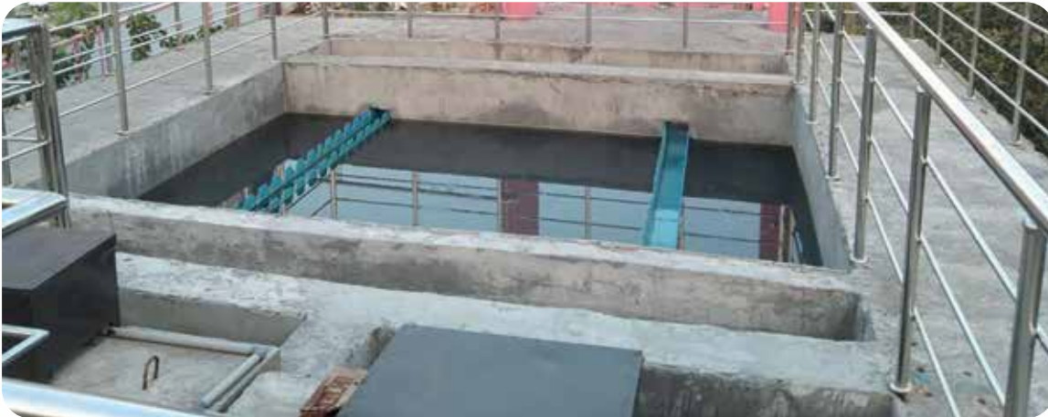
Effluent Treatment Plant of Space sweaters financed by Bank Asia Limited
