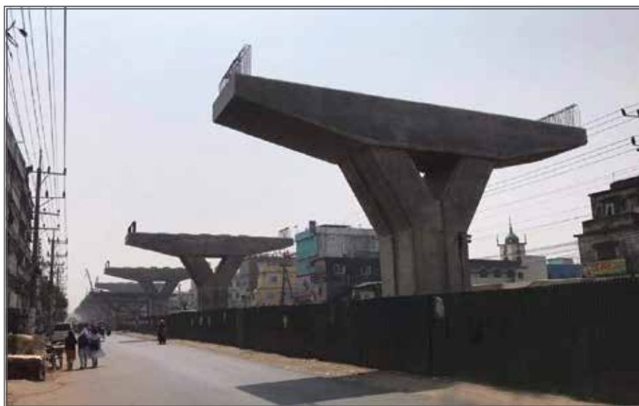
Bank Asia financed elevated expressway from Lalkhan Bazar to Sha-Amanat Airport, Chattogram
